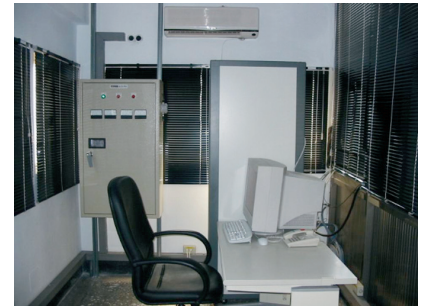
● 前端雷達站設備機房配置圖 A layout drawing of the front-end radar station equipment room
